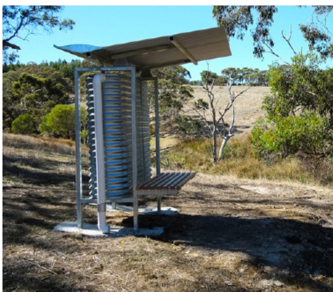
The water tank at Balquhidder is of steel construction. It was mandated by the Parks department.
